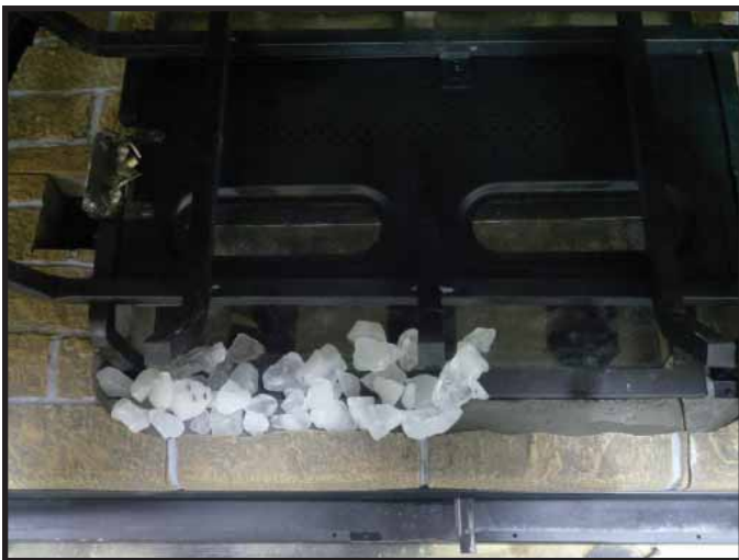
Figure 14.1. Install Teco-Sil
